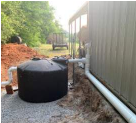
Photo – installation of a rainwater harvesting system in Nottoway (Dr. Gee)
