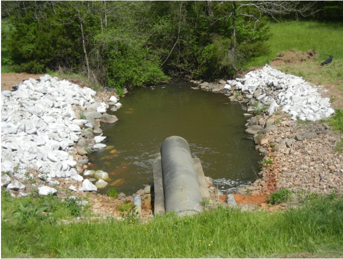
Outfall pool repair project after completion
