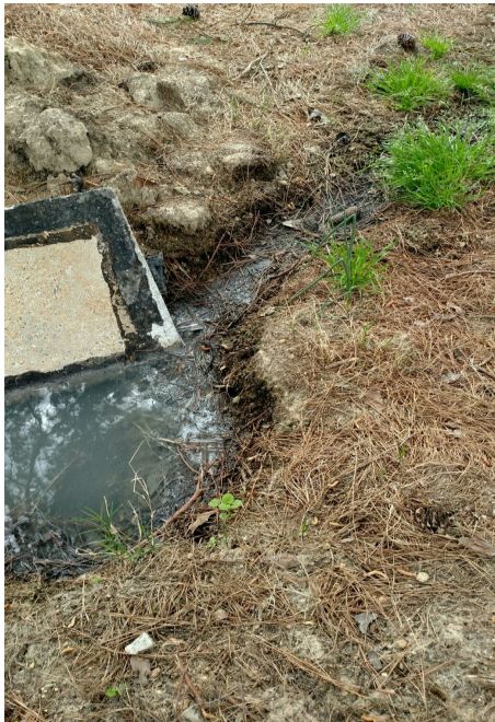
Failing septic system
