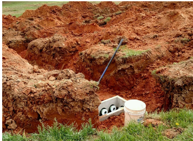
New drainfield of a repaired septic system
