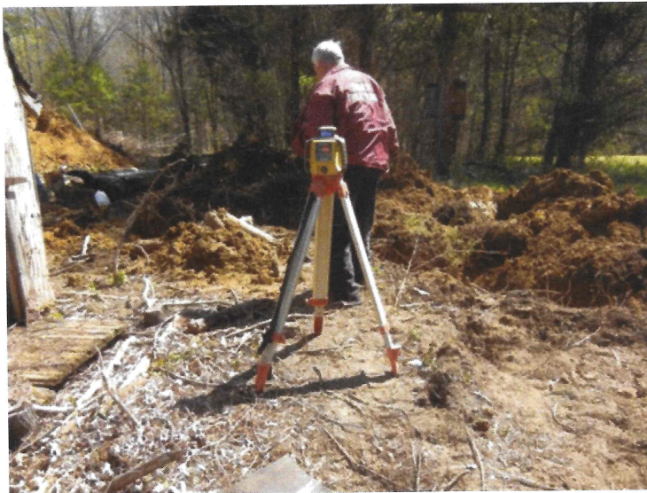
Some septic system repairs or installations require that the area is surveyed before any other work can begin.
